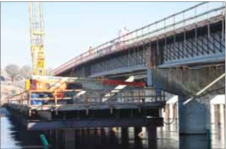
Work on the new north side of the Marsing Snake River bridge, shown in early November, is complete enough to shift traffic and start work on the south side.
