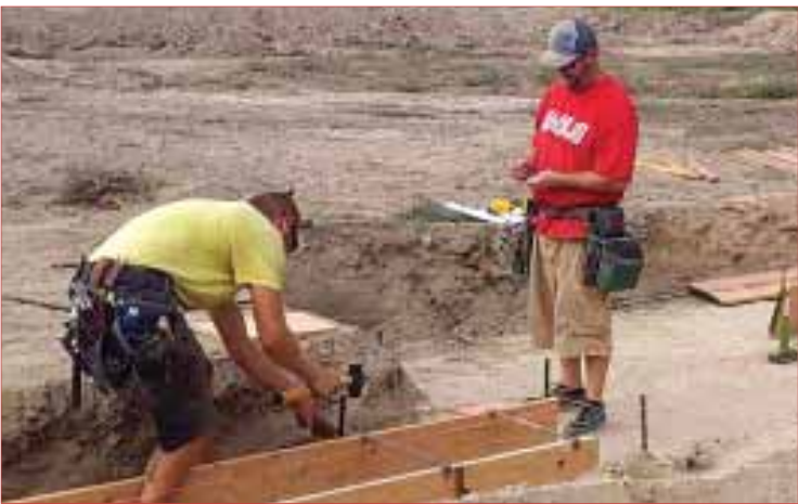
Employees from Ideal Custom Homes lay out forms in preparation for the pouring of footings to start construction of The Rock of Homedale teen center on East Owyhee Avenue. Submitted photo
