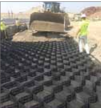
Above: An underground structure called a “geocell” was put into place before the roadbed was filled in. Left: Asphalt was then laid over. ITD photos
