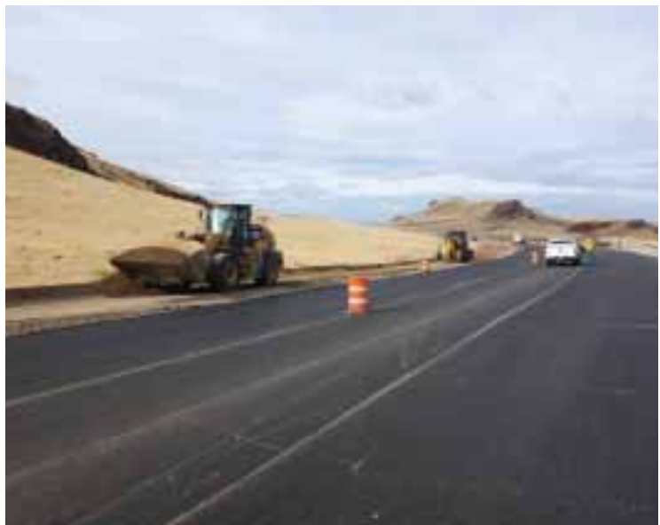
Above: An underground structure called a “geocell” was put into place before the roadbed was filled in. Left: Asphalt was then laid over. ITD photos
