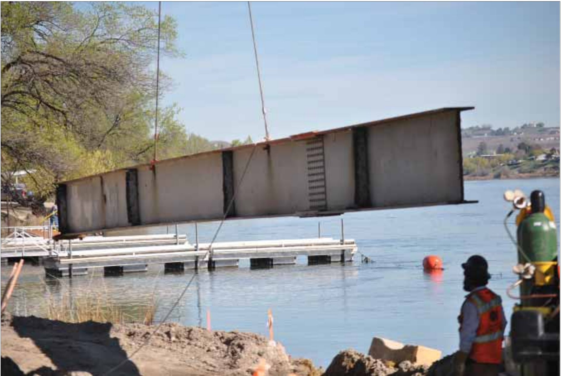
A crane lifts a large girder in Island Park during the beginning stages of demolition of the old Snake River bridge in Marsing. Demolition started last week and is expected to take three to four weeks.
