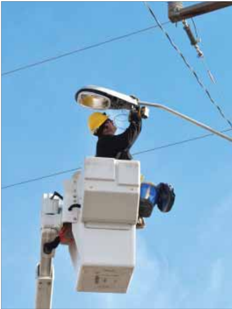
An Idaho Power employee installs a brand-new streetlight fixture with a 200-watt bulb at the southeast corner of Industrial Road and East Idaho Avenue. The work in February was part of several upgrades and new lights around Homedale schools.
