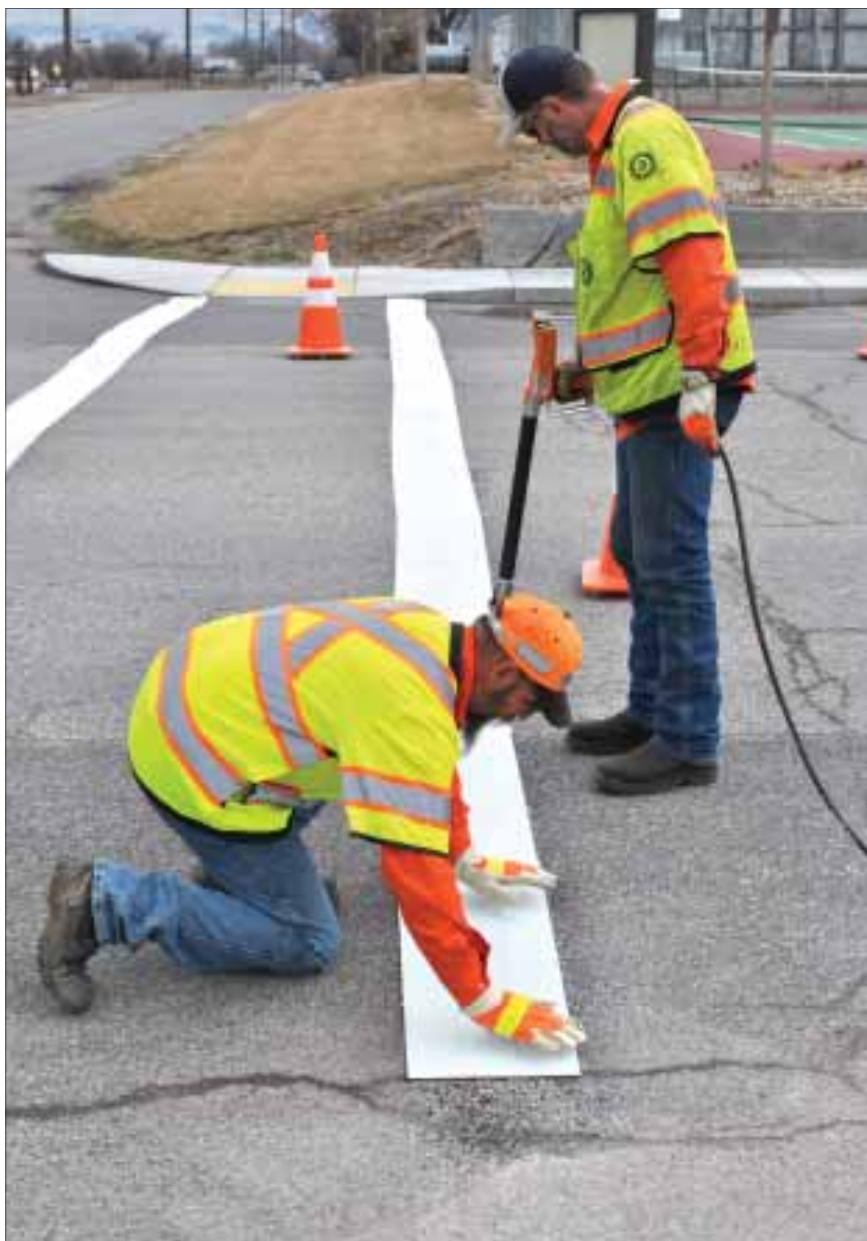
One Idaho Transportation Department technician puts down thermal-plastic crosswalk material while his partner uses a propane torch to heat it up and make it stick to East Idaho Avenue near the street's intersection with Industrial Road/North 3 rd Street East on March 6 in Homedale.
