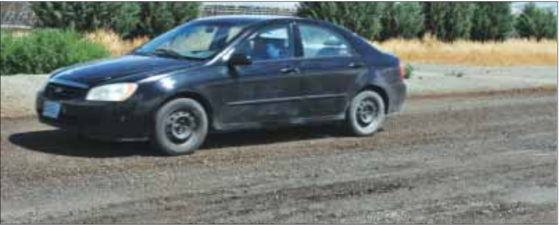
A vehicle travels a rotomilled portion of Johnstone Road, showing how a roadway treated with a sugar beet byproduct (above) reduces dust compared to untreated (left).
