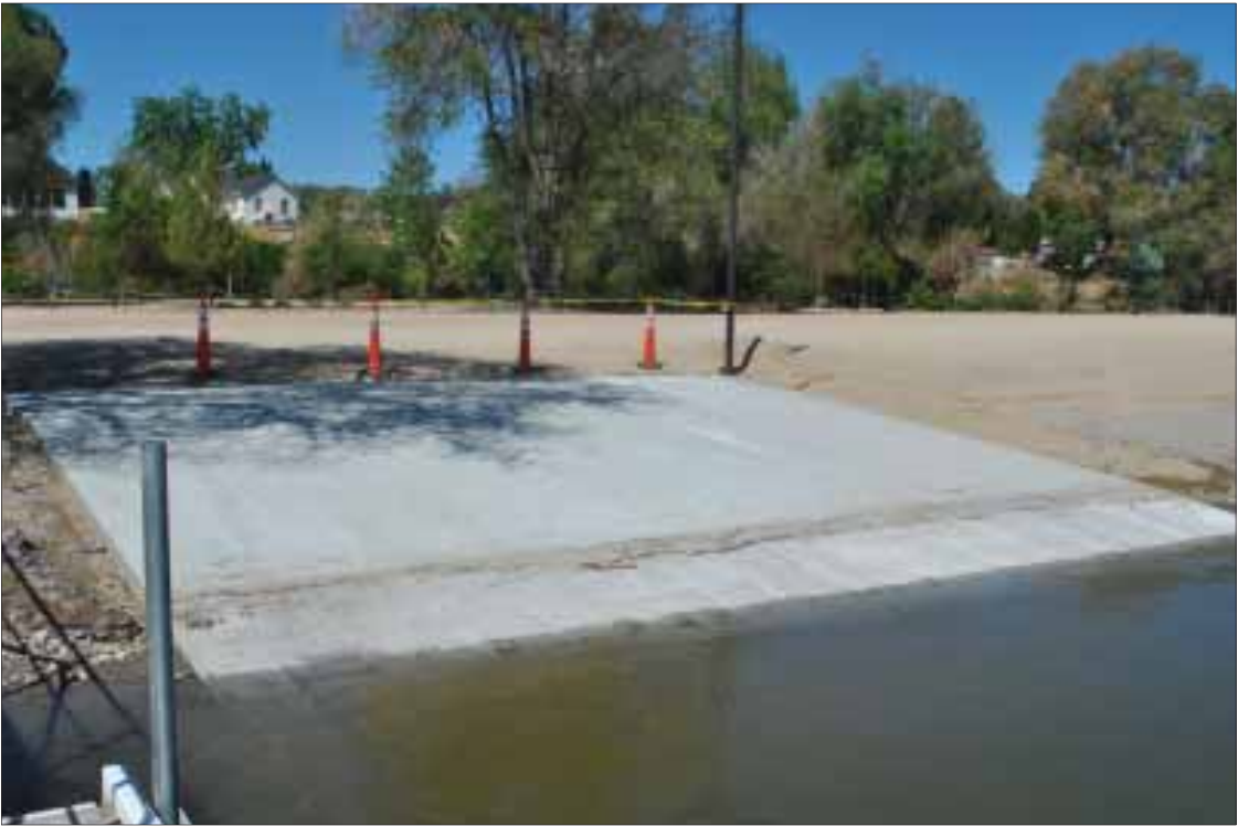
The upper half of the new Marsing Island Park boat ramp continues to cure on the bank of the Snake River.
