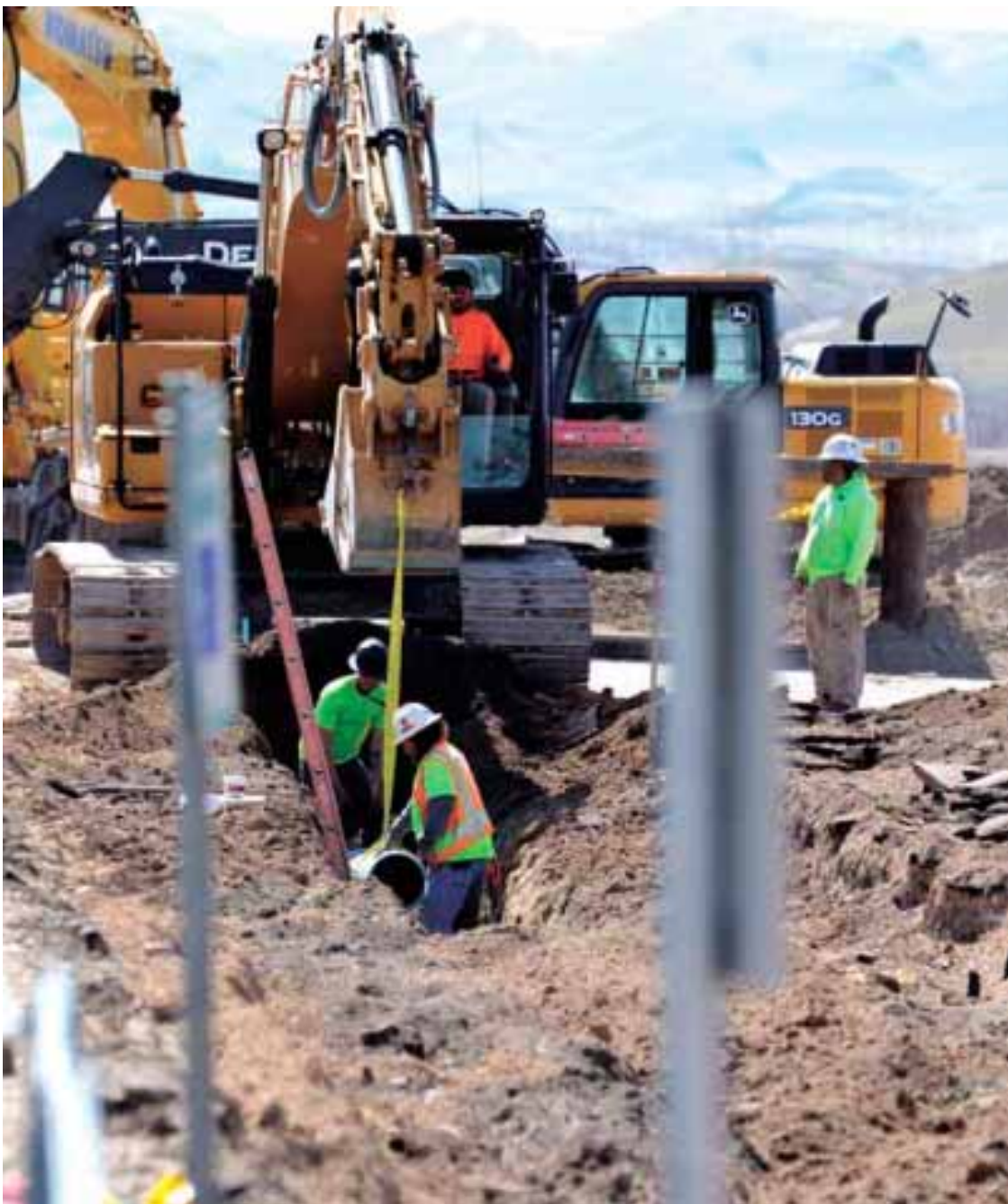
Workers laid down new sewer lines in front of the Marsing schools over spring break in preparation of the middle-school construction. The ground-breaking will be taking place at the site tomorrow at 2:30 p.m. The project is being spear-headed by Beniton Construction and Design West Architects.
