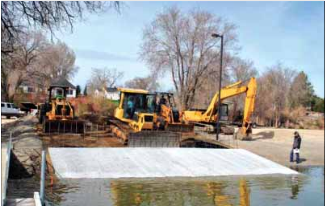
The concrete slab for the boat ramp gets pushed into the Snake River at Island Park last Thursday as Civil Dynamics' Kirby Cook looks on. Assisting with moving the slab are, from left, Marsing City's Ed Lowder, Precision Grading and Excavation President Gunner Bradford, and Marty McWilliams, an estimator for Precision.
