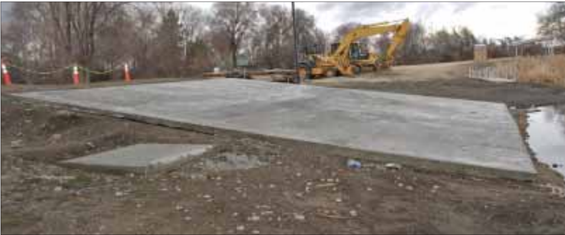
A cement slab for the new Island Park boat ramp sits ready to be installed in Marsing.
