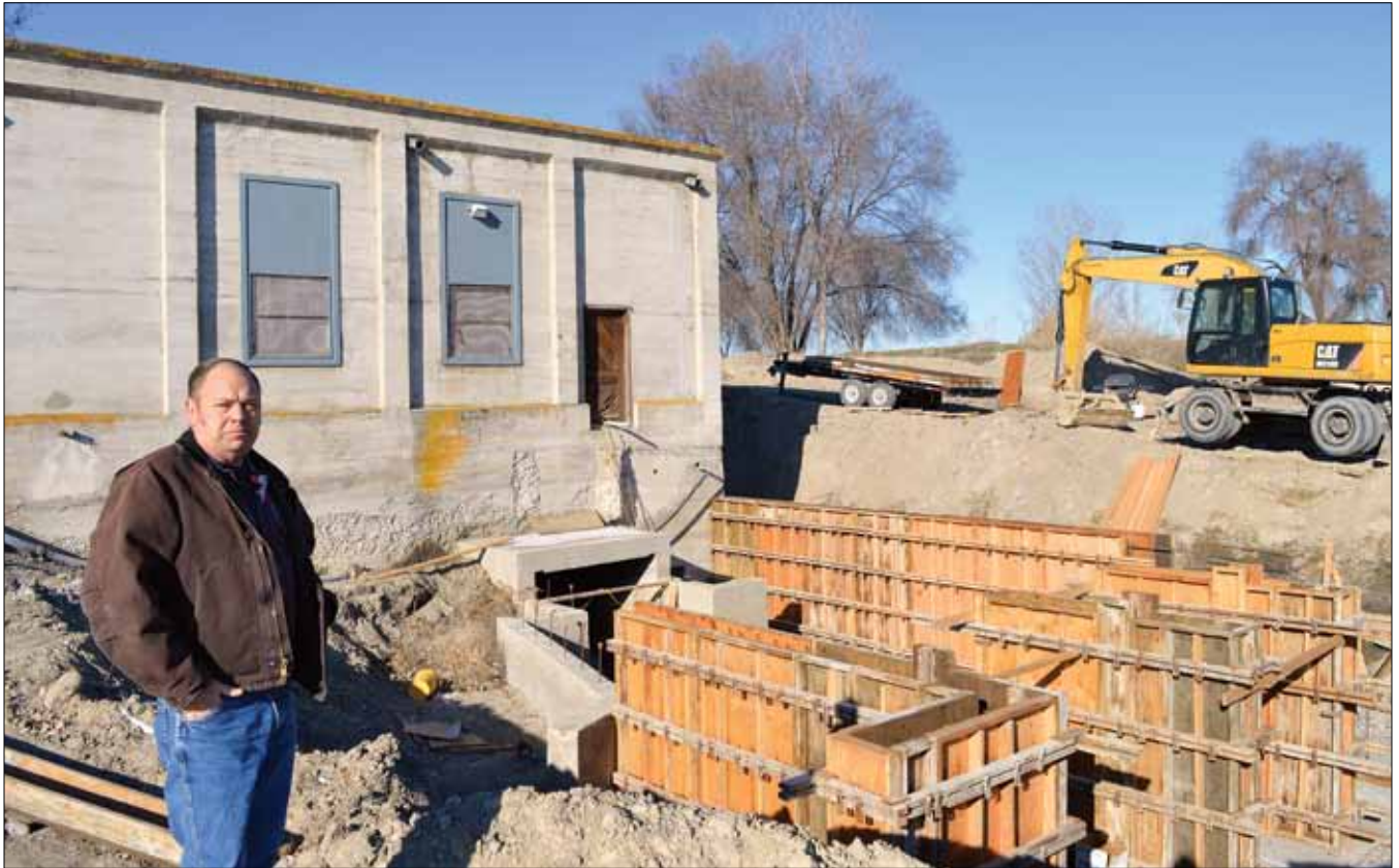
South Board of Control manager John Eells stands at the rear of the Gem 2 Pumping Plant on the Snake River near Homedale. The wooden forms were used to create a new concrete structure to replace large pipes through the Snake River flowed to the pumps.
