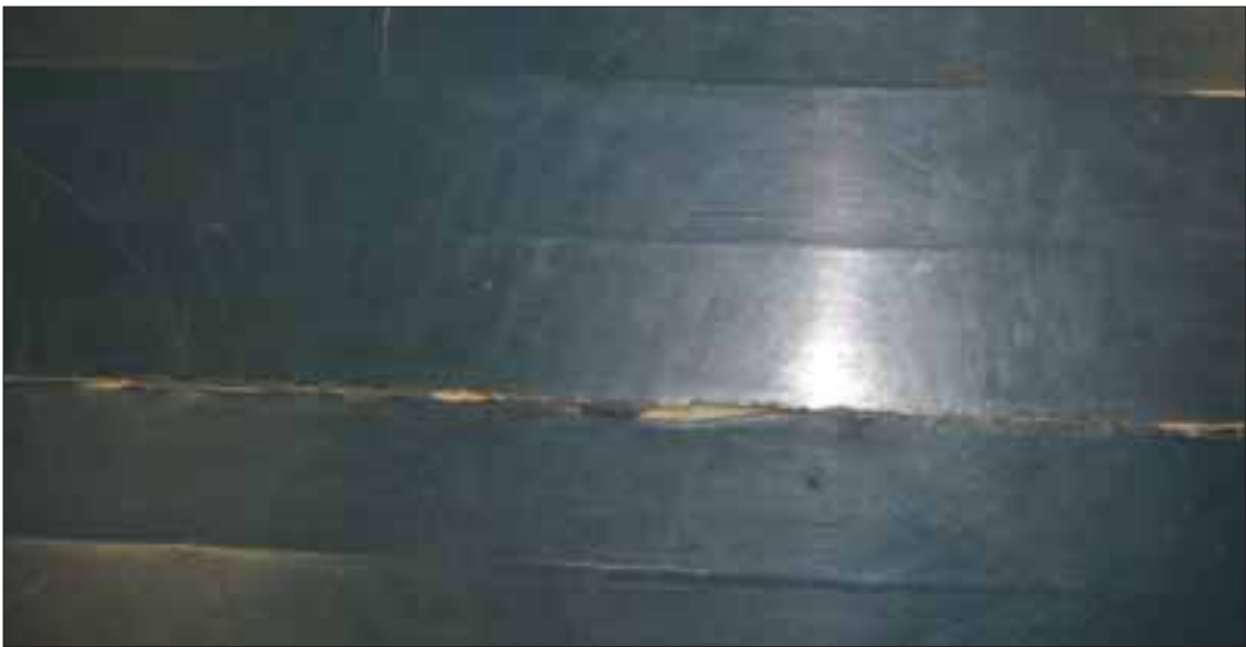
The Marsing High School gym floor shows some damage as a result of the broken pipe beneath the bathroom floor. There is some visible buckling and warping of the south side of the gym.
