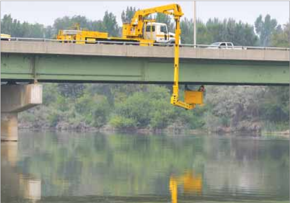
Two people in a boom lift bucket inspect the underside of the bridge spanning the Snake River outside Homedale last Wednesday afternoon. The work is done every two years on the bridge.
