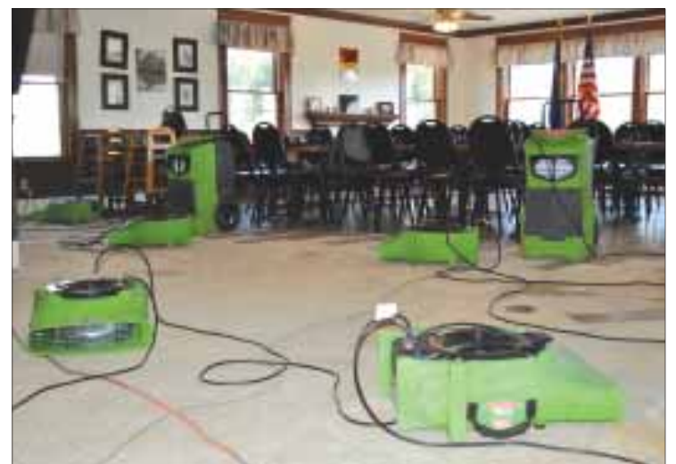
Industrial fans have been placed around the main dining room of the Sandbar to dry out subflooring damaged by a water leak that started last week.
