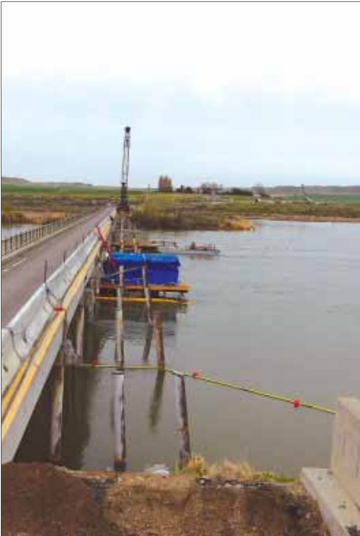
The approach for the demolished section of the Loveridge Bridge is seen next to the remaining old structure that is being used to ferry traffic across the Snake River outside Bruneau. Photo courtesy ITD
