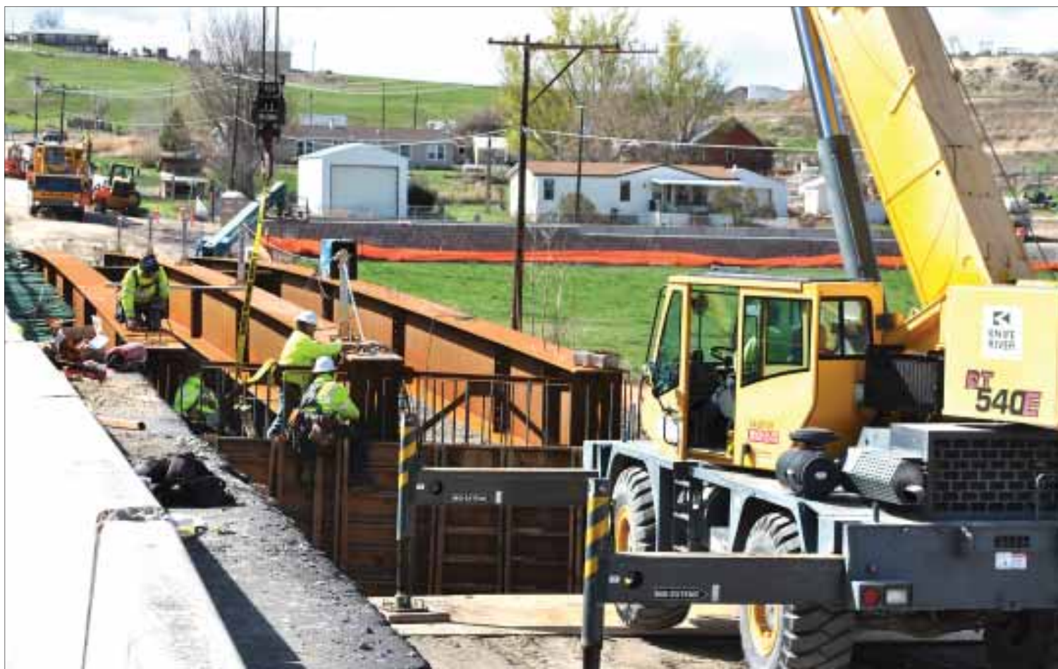
Knife River Construction crews place new girders on the north side of the Succor Creek Bridge in Homedale on Idaho highway 19. The March 27 work completed steel placement in the new span.
