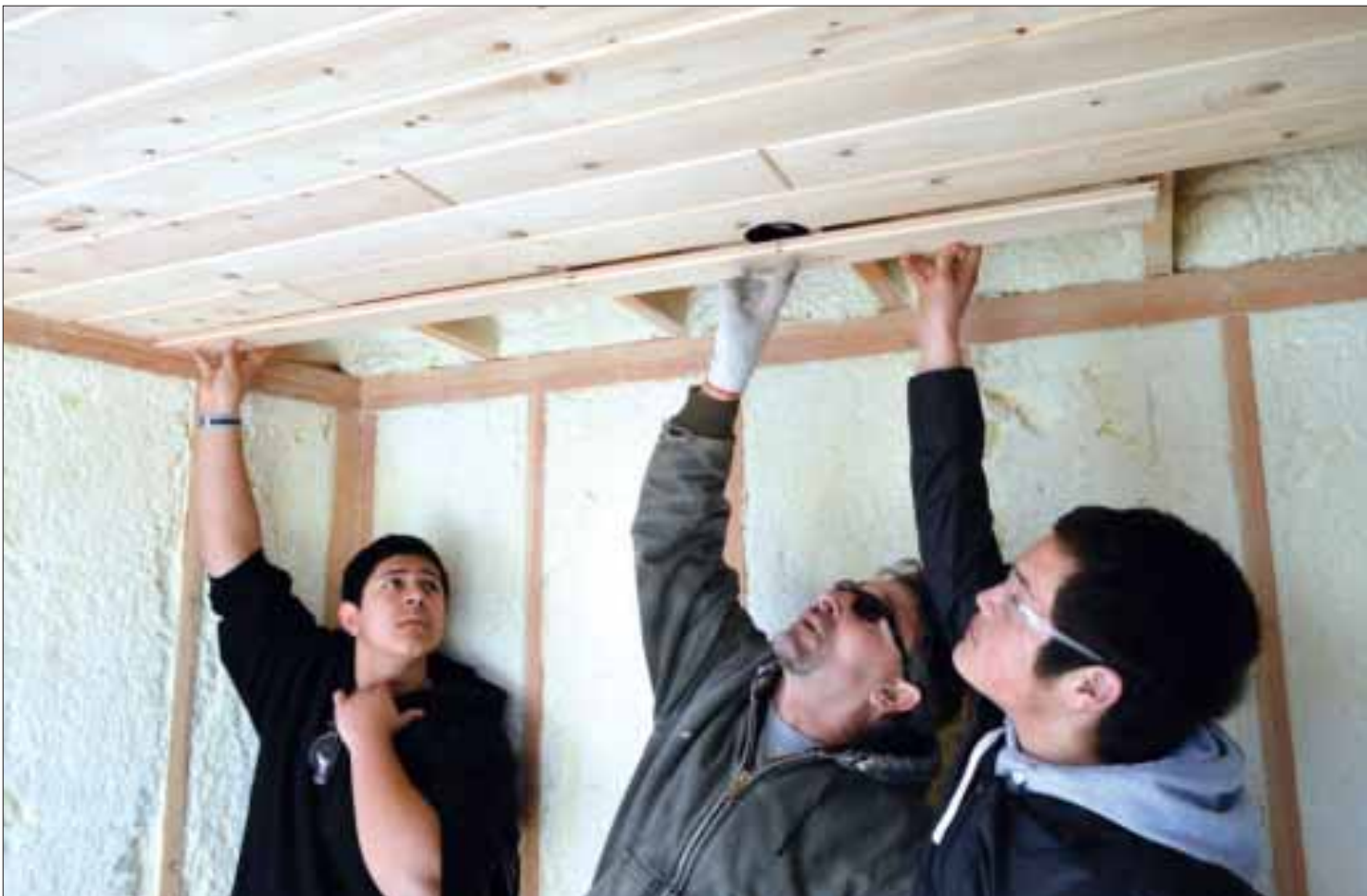
COSSA building trades instructor Rick Ray (center) shows Homedale High School students Angel Aviles (left) and Jose Buenrostro how to insert a slat into the ceiling above the kitchen area of the tiny house.
