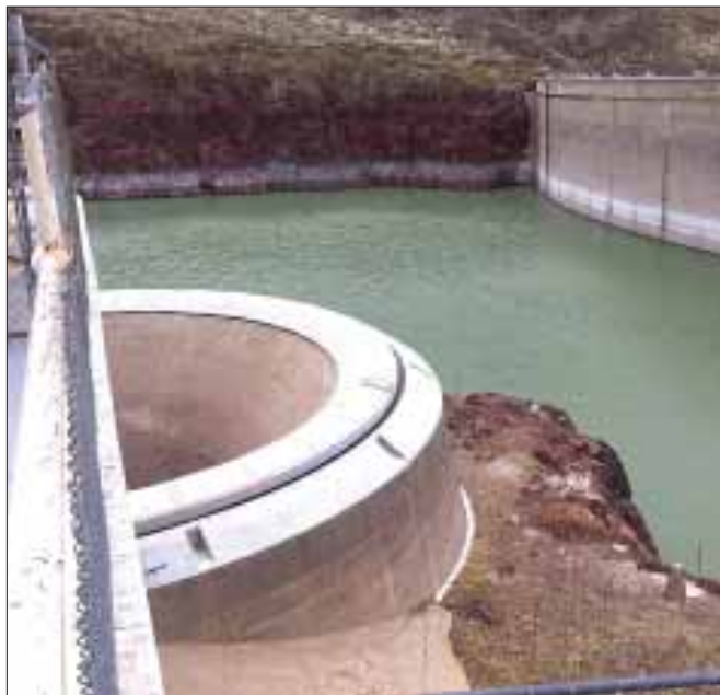
Left: The water level at Owyhee Reservoir was so low on Jan. 30, 2016 that the outcropping below the dam's ring gate was visible as was the water line on the dam and shoreline. Right: On Feb. 25 this year, the lake's level was much higher, and the ring gate could be in operation for the first time in six years. Photos by Dave Downum
