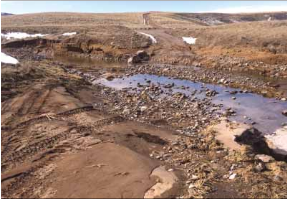
Recent runoff caused erosion that washed out the Saylor Creek Crossing in the Jarbidge Field Office of the Bureau of Land Management Twin Falls District. BLM photo
