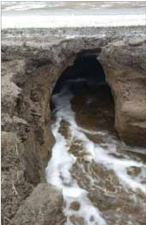
Water rushes through a gaping hole that developed under the roadway on Idaho highway 78 last week. ITD photo
