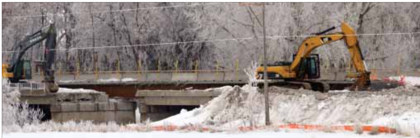
Workers and heavy equipment from Qualitree operated in frigid temperatures Friday to continue demolition of the old Idaho highway 19 bridge across Succor Creek west of Homedale. A girder of the new eastbound span was exposed after a section of the old bridge was destroyed earlier in the week. A worker tries to manipulate a tangle of concrete reinforcement bar.
