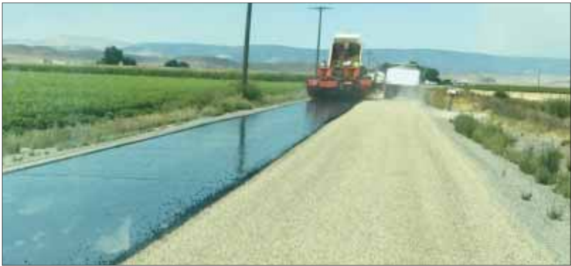
A Homedale Highway District maintenance crew was busy chip-sealing a section of Graveyard Point Road on Monday.
