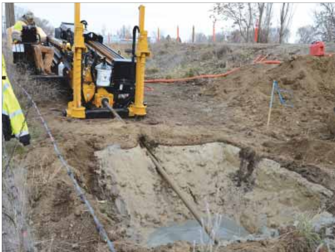
A Warrington Construction technician bores pipe into the embankment near the Succor Creek bridge.
