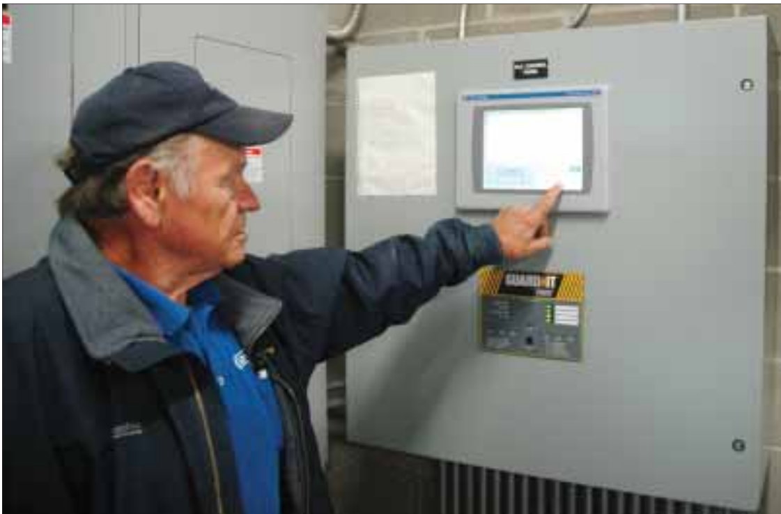
John Larsen explains how the Marsing methane gas recovery project's control panel works to track pressure in the methane containment dome, generator status, and water tank level.
