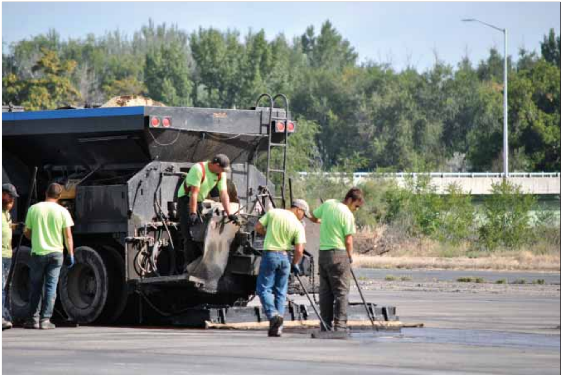
A crew from Eugene, Ore.-based Pave Northwest spreads slurry seal during a runway rehabilitation project at the Homedale Municipal Airport last Wednesday.
