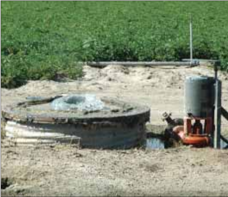
Irrigation water flows out of bubbler near an agricultural field northwest of Homedale.
