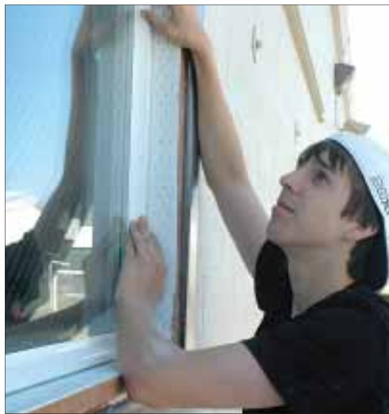
Kyler Landa studies a safety window frame to ensure it is lined up correctly during installation at the Homedale High School gymnasium.
