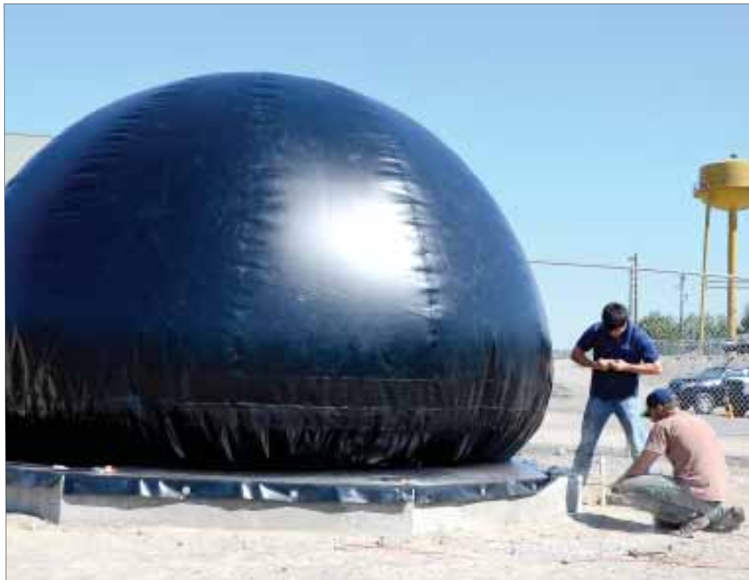
Grady Turner, left, and James Schroeder of DC Engineering installed the new methane storage tank in Marsing last week. Photo by Karen Bresnahan
