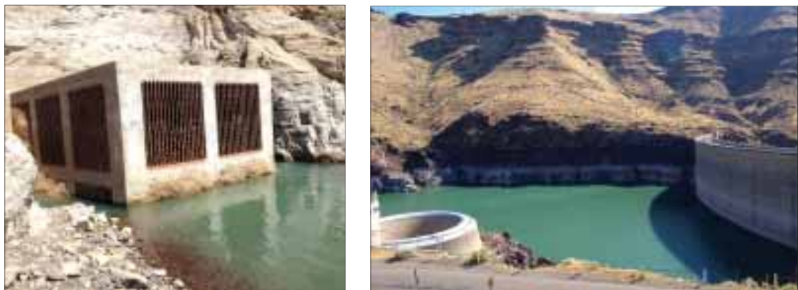
Another low-water year has exposed structures not usually seen at the Owyhee Reservoir. Left: The irrigation inlet. Photo by Mark Aman Right: The glory hole near the dam. Photo by Vern Tunnell
