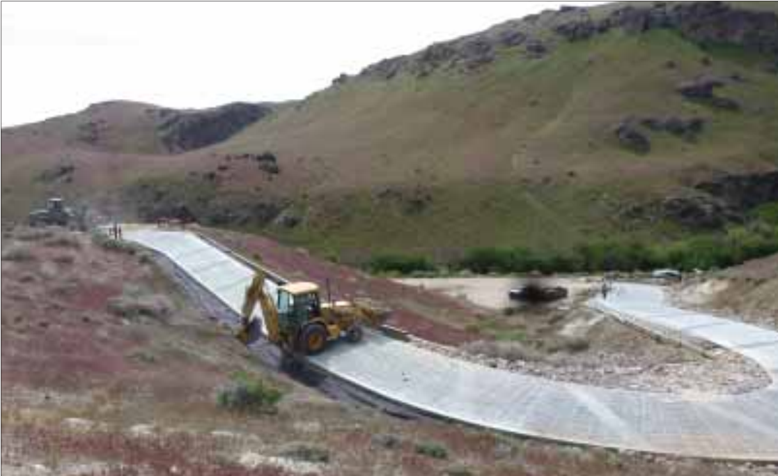
Above: BLM crews and heavy equipment worked on reconstructing and laying concrete down on Jump Creek Recreation Site access road this spring. Below: Prior to the project, the road was steep and lacked drainage. BLM photos
