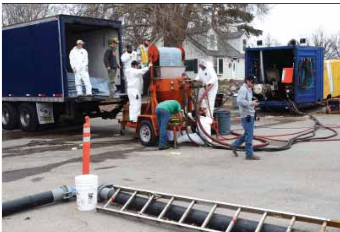
Workers from the Pipeline Inspection Services Inc., begin work on a manhole in the northeast section of Marsing. The men are putting in new slip lining by blowing a sock liner inside the piping and using heat and cold to cure the product. Total cost to the city was around $159,000, and the project was supposed to be completed earlier this week. Photo by Karen Bresnahan
