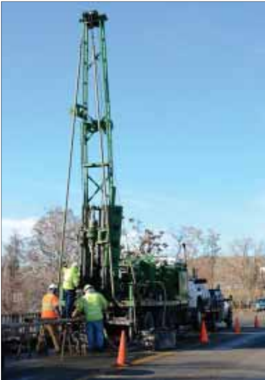
Crews from Meridian's Haztech Drilling and Boise-based Terracon Consultants work on soil testing procedures at the Succor Creek bridge west of Homedale on Idaho highway 19. Photo by Karen Bresnahan
