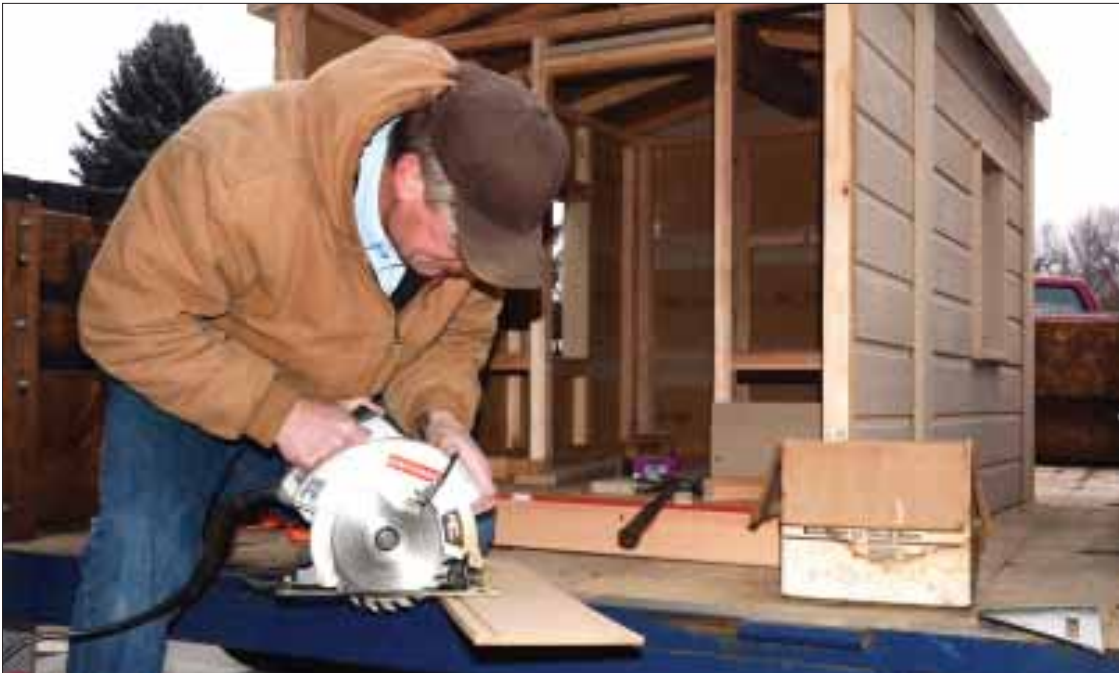
Larry Cooper uses a circular saw to cut siding for the miniature house. Photo by Karen Bresnahan
