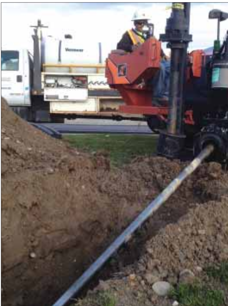
Above: Alberto Gonzaga of Track Utilities Inc., of Meridian, bores a hole through which route electrical wiring will be routed to the Welcome to Homedale sign location. Below: Homedale assistant public works supervisor Bret Smith, center, stands with Uria Pump owner Ric Uria, left, and Track Utilities' Cristian Manriquez Submitted photos
