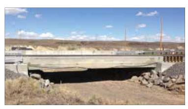
A new concrete slab bridge replacing worn-out culverts under Idaho highway 78 at Scorpion Creek is now open to traffic in both directions. ITD photo
