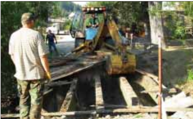
Silver City bridgework finally starts An Owyhee County Road and Bridge crew began work Aug. 26 to replace the deteriorated wooden bridge across Jordan Creek in Silver City. Work should be completed by the middle of the month. Photo by Clarence Orton
