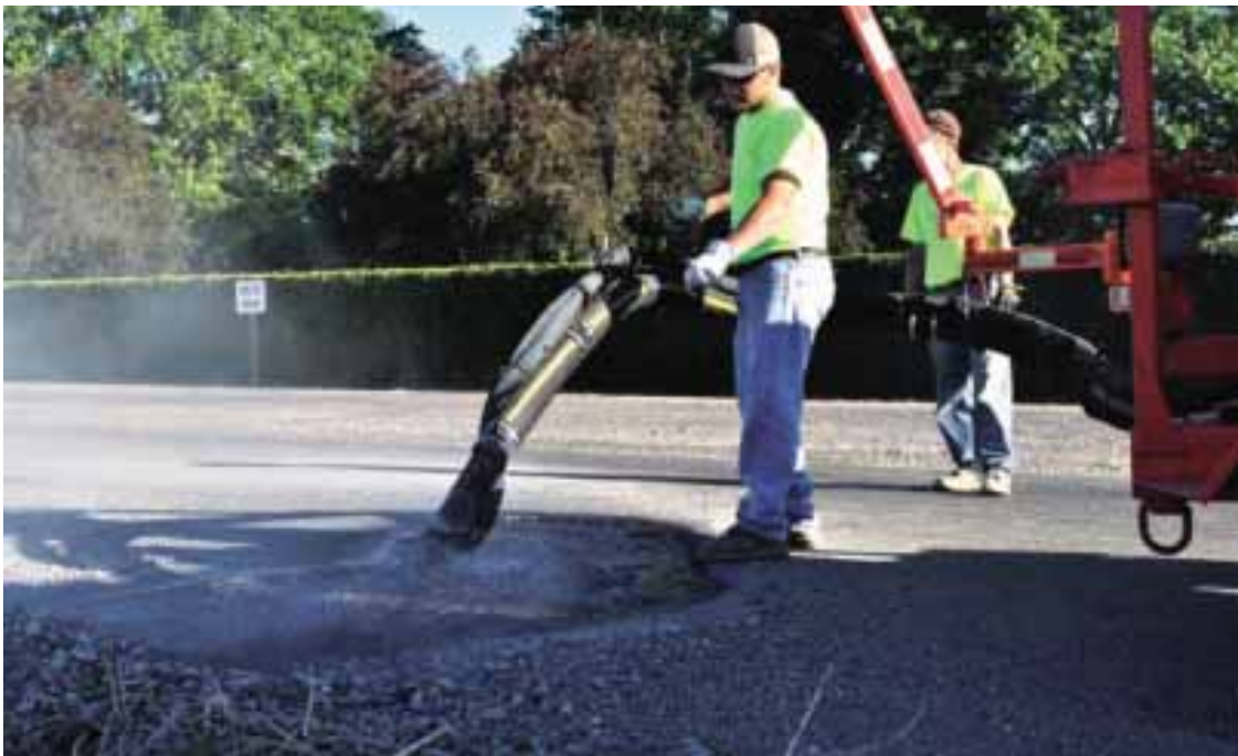
Homedale Highway District assistant director of highways Dan Herman uses the DuraPatcher to spray aggregate on Cemetery Road as director of highways Stuart Constantine watches for passing vehicles.
