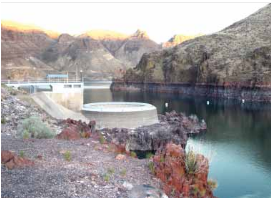
The Owyhee Reservoir water level is low enough to expose a good portion of the glory hole near the dam. Photo by Lori Bahem
