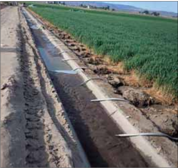
Above: South Board of Control and some local farmers have developed silt ponds to reduce the amount of sedimentation building up in irrigation ditches after water runs off fields. Left: Silt build-up clogs a ditch in the South Board of Control region, backing up water destined for a furrow-irrigated field. Submitted photos
