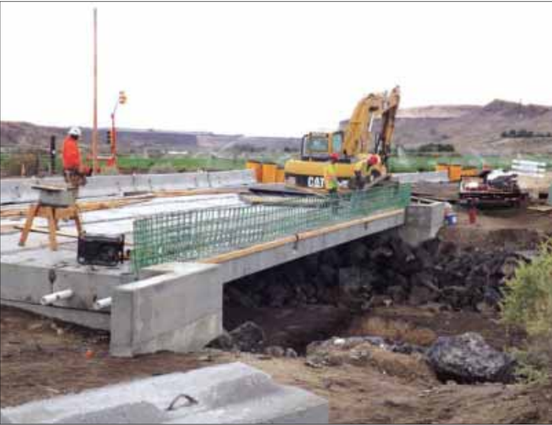
Knife River Corp. Northwest employees continue work on the concrete slab bridge that will carry Idaho highway 78 across Scorpion Creek. ITD photo
