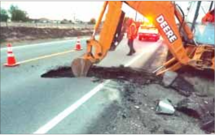
An emergency road repair crew from the Idaho Transportation Department went to work on a sinkhole that comprised Idaho highway 78 outside of Givens on May 6. ITD photo
