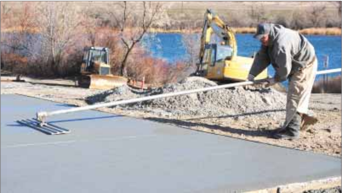
Buck Peak, who works for the Idaho Fish and Game engineering department, smooths cement at Bernard Landing during December construction.
