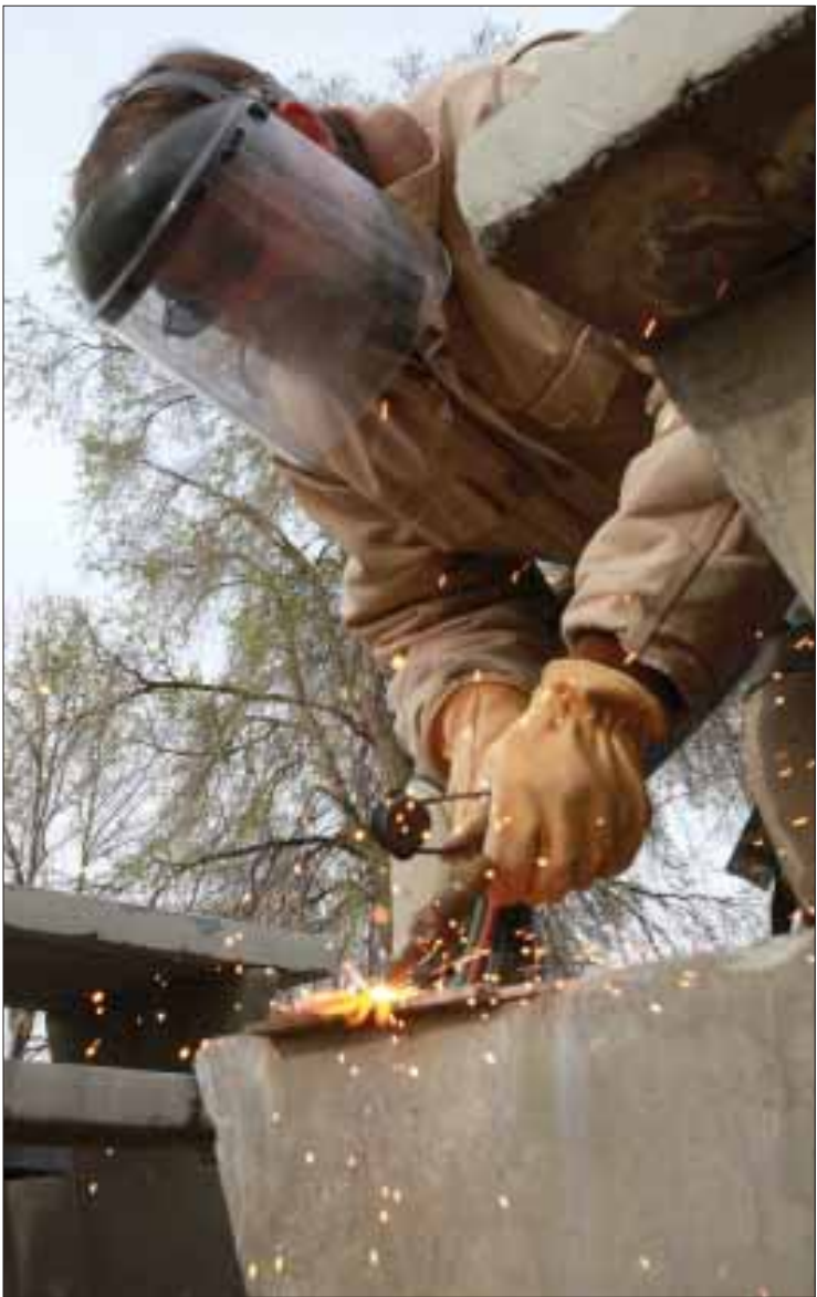
Ray Jensen uses a cutting torch to remove old bench supports on the concrete picnic tables at Bette Uda City Park on Friday in Homedale.
