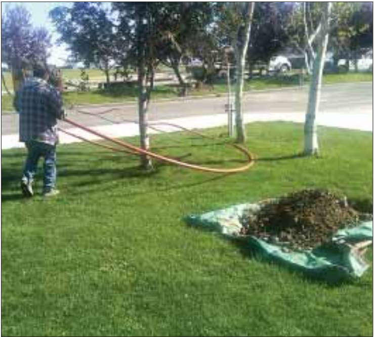
A worker moves innerduct piping used to house fiberoptic cable at Homedale Middle School during last year's project.
