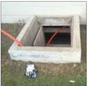
Innerduct runs into the crawlspace of Homedale Elementary School. Submitted photos
