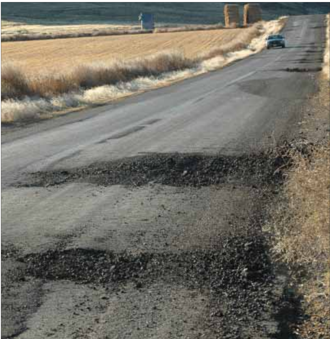
A vehicle on Monday morning navigates numerous potholes caused by heavy trucks that travel on Nielsen Lane south of Graveyard Point Road.
