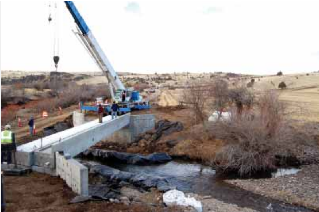
Construction workers from Payette-based Braun Jensen Inc. place concrete and steel girders at the site of the new Jordan Creek Bridge on Flint Creek Road in December. Photo by Matt Hall / HMM Engineering.
