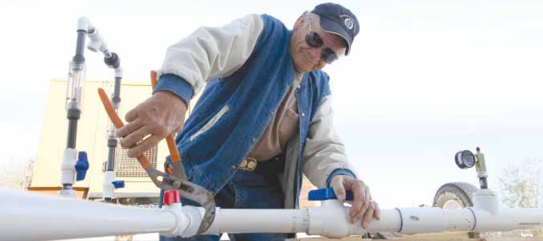
Marsing's methane project manager John Larsen puts the finishing touches on a test collection unit used to pipe captured methane into a 30kW generator at well No. 1.
