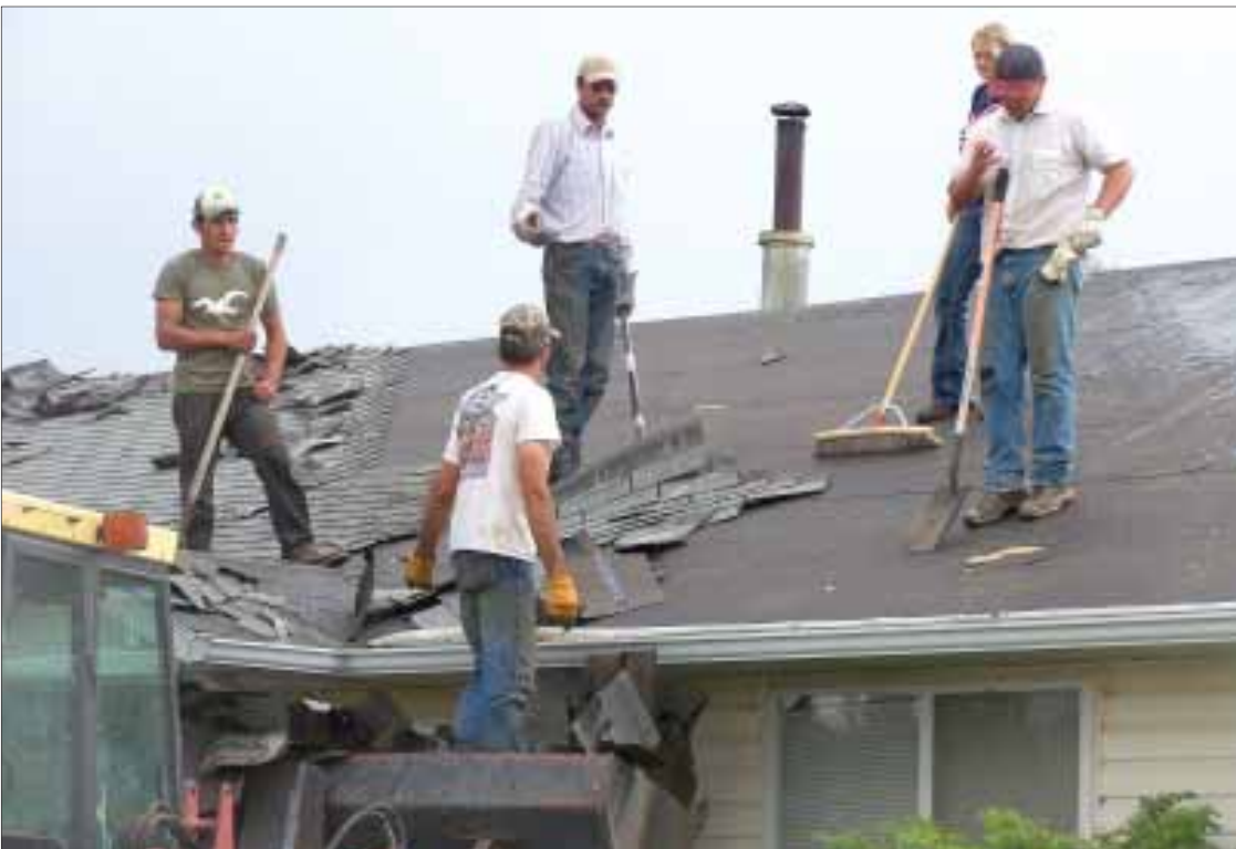
Above: Volunteers clear away shingles from the roof of the Pleasant Valley School. Below: Volunteers take the roofing down to the wood and work their way across the schoolhouse roof. Submitted photos
