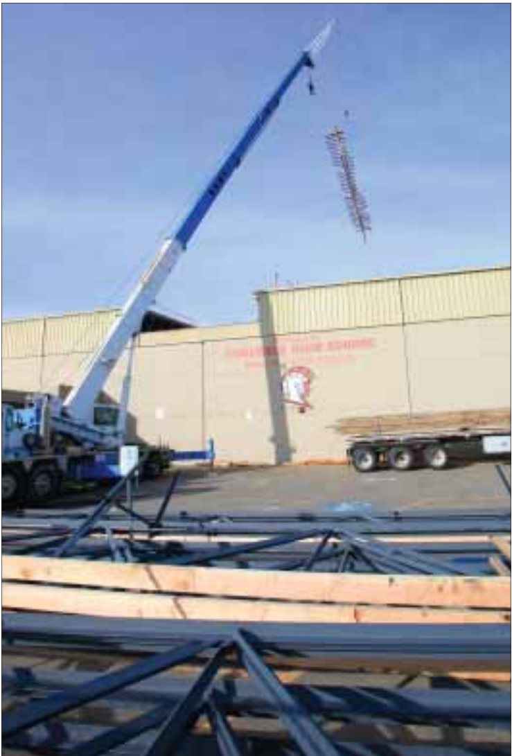
A crane operator carefully removes one of the old wooden trusses from the Homedale High School gymnasium last week. Construction crews removed the old beams and installed the new ones throughout the week.
