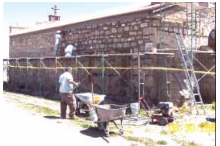
Left to right: Mackie Landon, Eric Smith and Fred Abritz from Kuna-based Budd Landon Masonry apply new mortar into the native stones on the south wall of the Our Lady Queen of Heaven Catholic Church in Oreana. Submitted photo
