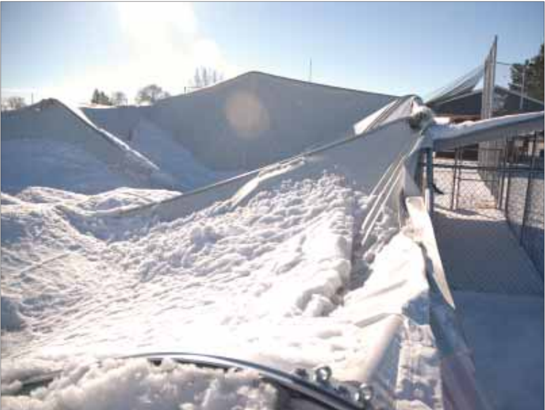
The awning between fields 1 and 2 at Sundance Park collapsed during overnight Thursday under the weight of snow that accumulated in Wednesday's storm.
