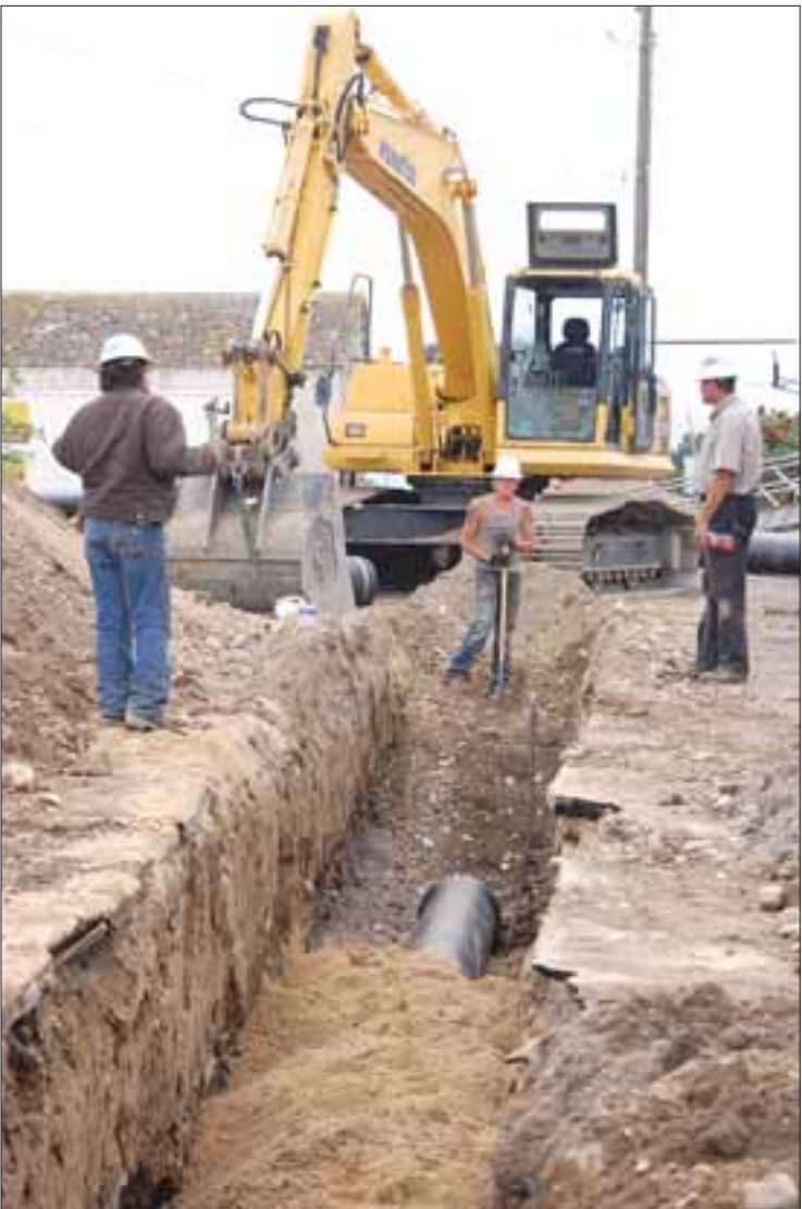
A crew installs a pipe beside Main Street in Marsing last fall. It was part of more than 12,000 feet of new water lines buried throughout the city.
