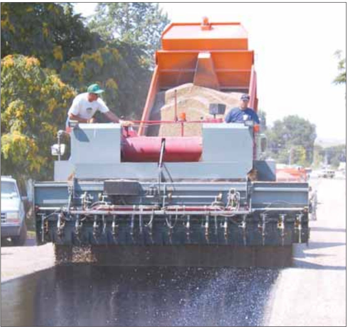
Chip seal Crews coat oil on Homedale streets last week during a seal-coating project. Homedale maintenance supervisor Larry Bauer said the project was a one-day project.
