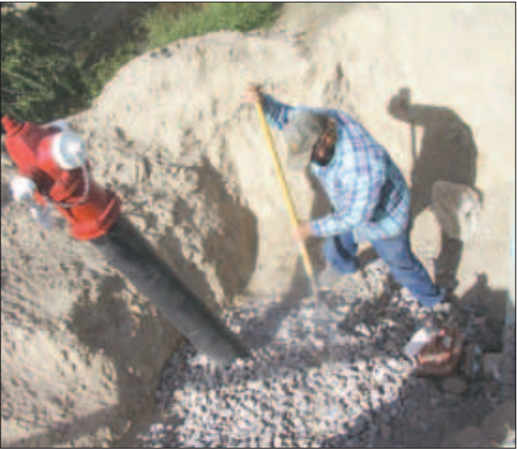
Emergency water line Homedale City Maintenance worker Scott Mahler installs a fire hydrant at the end of the Snake River Bridge near Homedale last week. Maintenance crews have been installing a water line across the bridge to continue uninterrupted water service to the city as the city's main water line is repaired. The city council passed an emergency funding of the project last month after City Engineer Bob Walker voiced concerns that the line could break and could possibly cause sever damage to the bridge.
